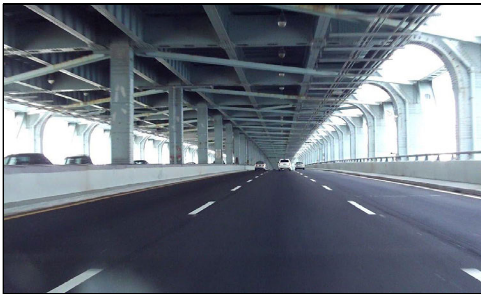
Figure 3-4: Lower Level Suspended Span
