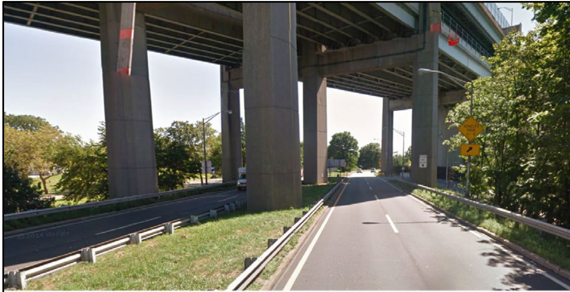
Figure 5-11: Limited Width Due to Brooklyn Ramps under the VNB near the Anchorage
