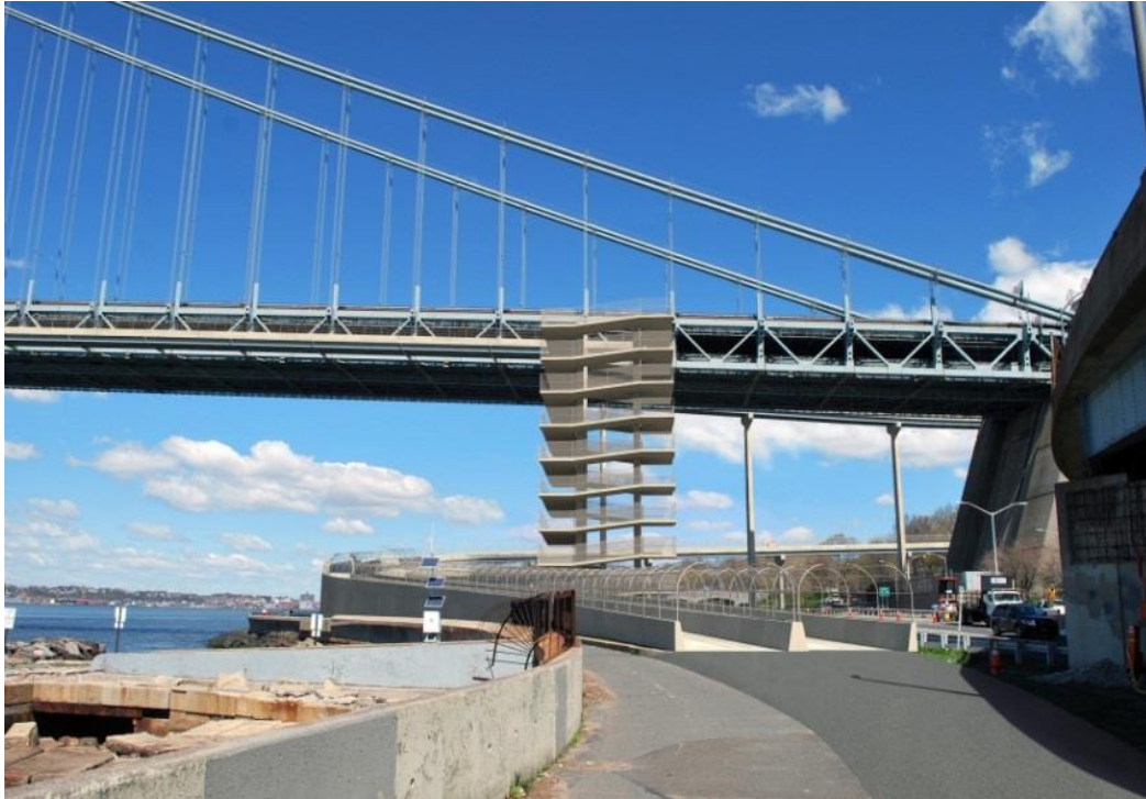
Figure 5-3: Lower Level Outboard Shared-Use Path – Brooklyn Pedestrian Ramp Access
